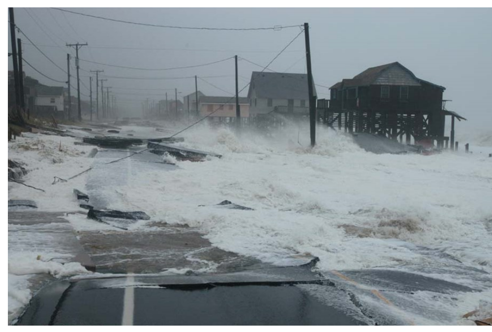
Destruction due to wave run-up and wave overtopping
