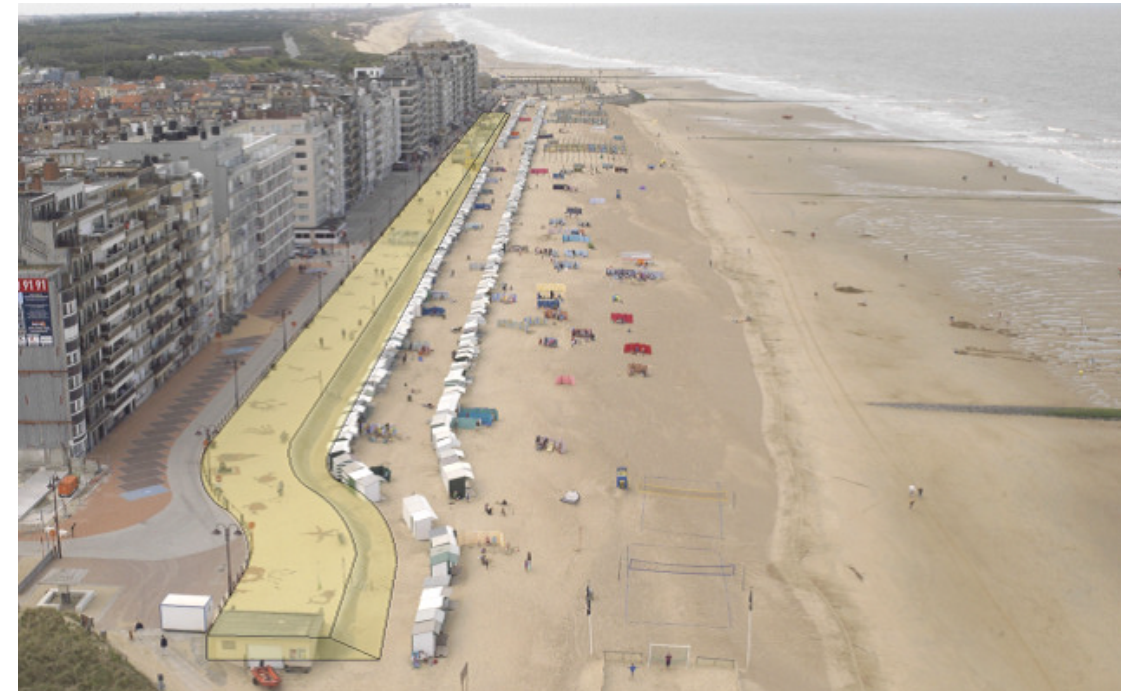
Typical situation at the Belgian coast. Foreshore, dike and promenade (source: W. Vaele)
